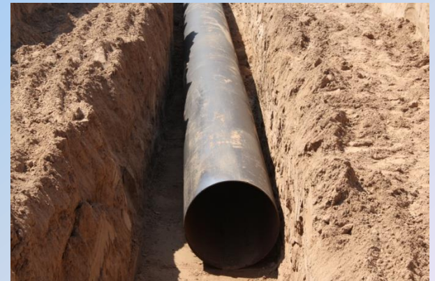
Grade Stabilization Structure (410)
